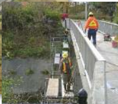
City of Kitchener Bridge Rehab
