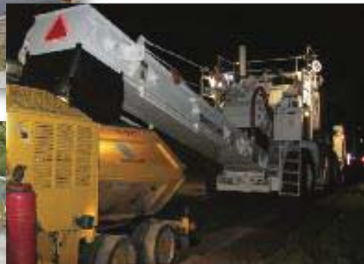
Hwy. 7&8 BOT Paving
