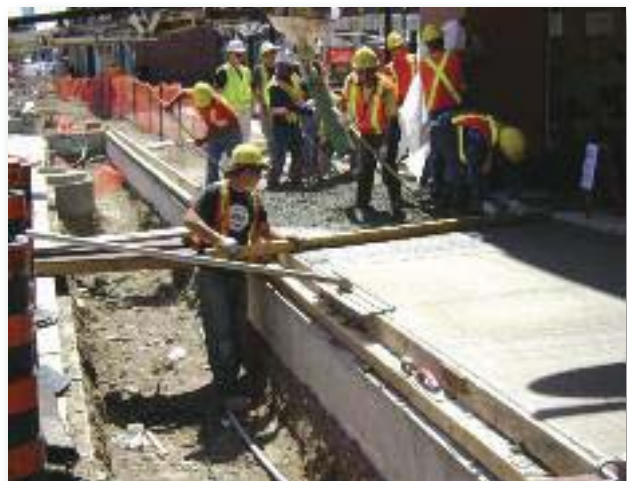
King St. planters & sidewalk
