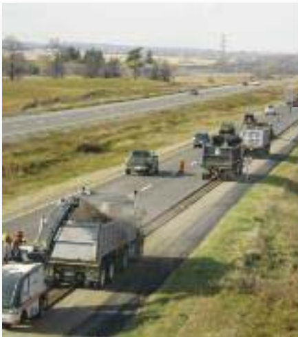
Hwy. 7&8 partially paved shoulders
